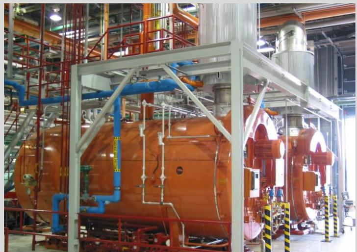
Four steam gas boilers (natural gas, oil backup): 73 000 lbs/hr, 2200 hp, 50 to 125 psi. Enough energy to heat about 1000 average homes for one year. Used for heating, humidification and the production process.
