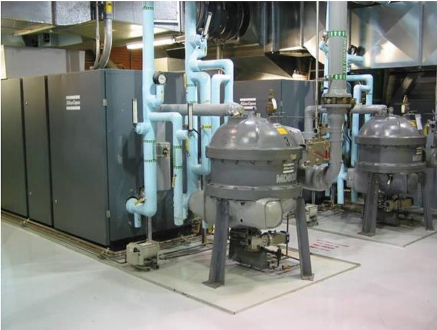
The Bromont plant replaced a vacuum system that used air compressors with a central vacuum system.
