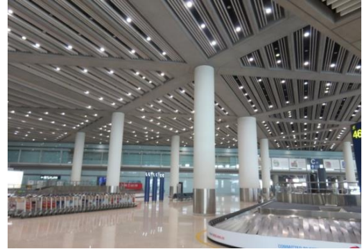
Figure 6 T3 lighting system
