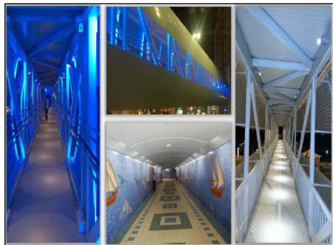
Photo No. (3): Smart Lighting (LED Lighting) in some Pedestrians Bridges in in Abu Dhabi City
