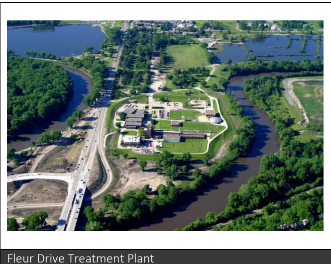
Fleur Drive Treatment Plant
