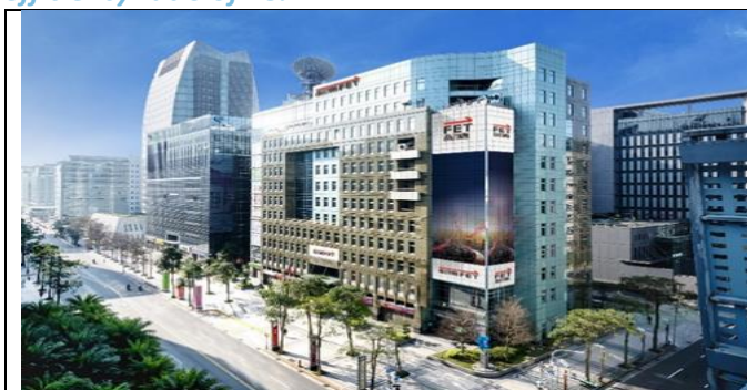
Far EasTone Telecom Headquarters (Office/IDC)
