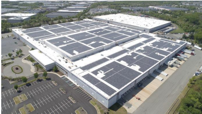
Figure 1: IMDC 7.2 MW solar installation, Edison, NJ
