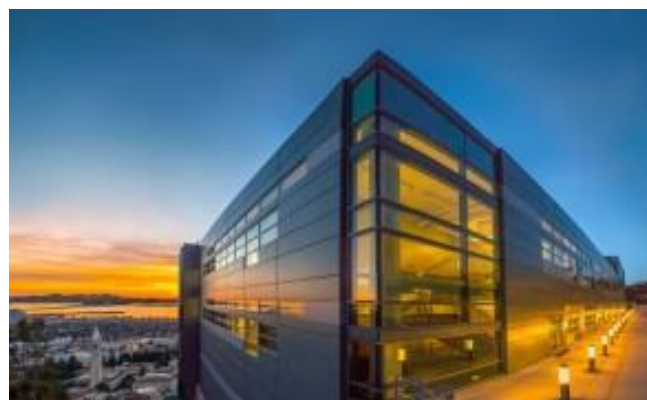
Berkeley Lab's Shyh Wang Hall is a LEED-certified gold building that houses the National Energy Research Scientific Computing Center (NERSC).
