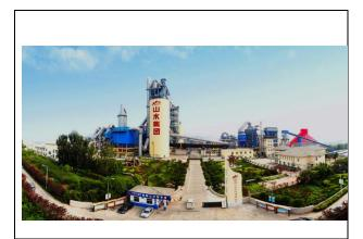
Linqu Shanshui Cement Co. , Ltd. has two new dryprocess Rotary Kiln clinker production lines with a daily output of 4000 tons and a 16.5 mw pure lowtemperature waste heat power plant and a cement grinding production line with an annual output of 1 million tons
