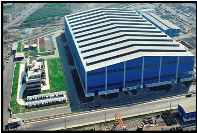
L&T-MHPS Turbine Generators-Aerial view
