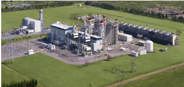
C. T. Genelba Power Plant
