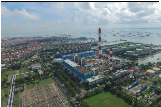
Gresik Power Station
