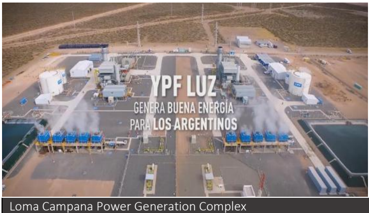
Loma Campana Power Generation Complex
