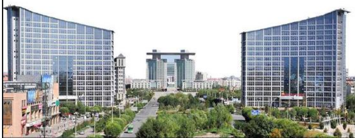
Yumen Oilfield Production Command Center.
