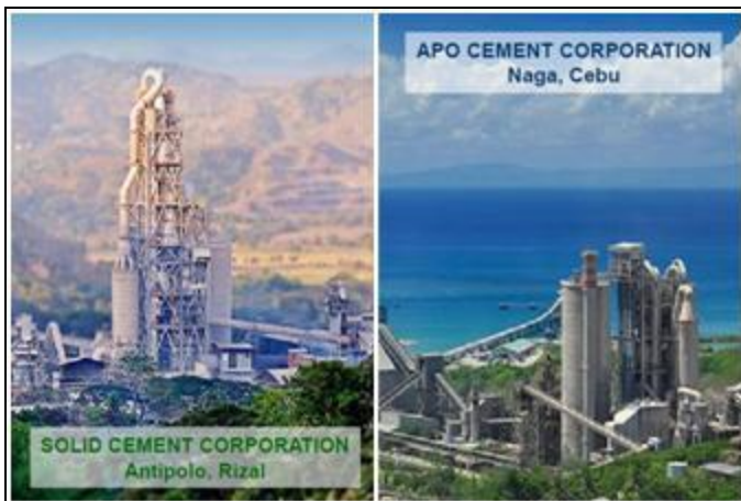
Figure 1. Aerial shot of the two CEMEX cement plants in the Philippines
