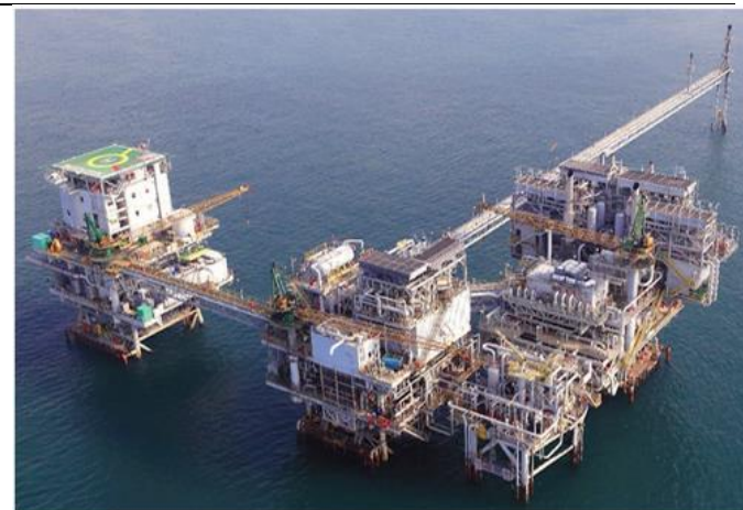
Mike Mike Flow station; one of PHE ONWJ's offshore facilities
