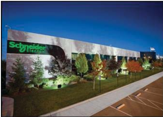
Figure 1 - Schneider Electric's Clovis, CA Facility – an ISO50001 and SEP Platinum certified facility
