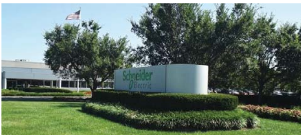
Figure 9 - Schneider Electric's Lexington, KY Plant - an ISO50001 certified and SEP Silver facility
