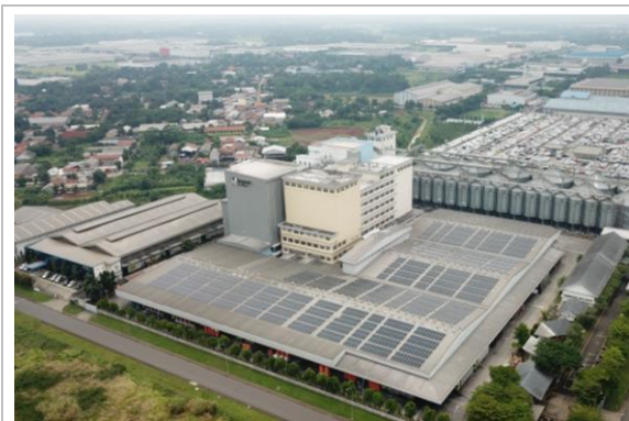
Figure 5. Clean Energy - Solar PV Application
