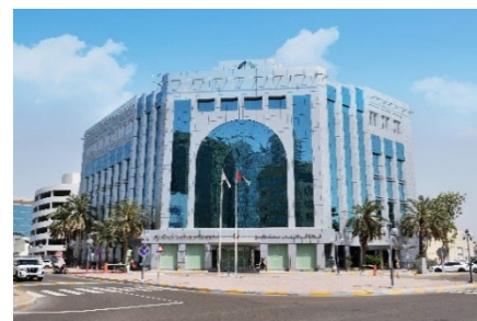
Figure 1: ADDC’s HQ in Abu Dhabi
