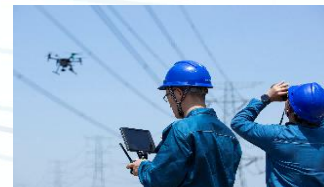
UAV Inspection for Power Lines
