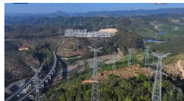
China-Laos 500 kV Interconnection Project
