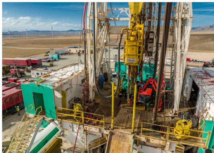
Drilling operations at the Utah FORGE field laboratory, showcasing advanced downhole tools and well construction technologies. Source: Flash Point
