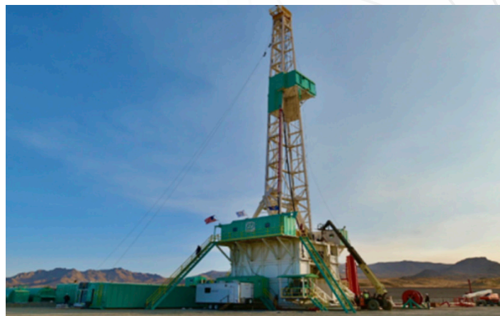
Drilling rig at the Utah FORGE field laboratory in Utah, supporting deep drilling and reservoir stimulation. Source: Eric Larson
