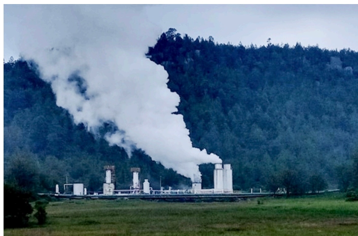
Los Azufres geothermal power station. Source: CFE
