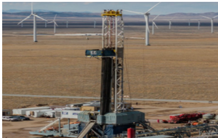
Advanced geothermal drilling operations. Source: www.capestation.com
