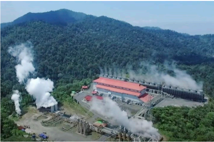
Salak Geothermal Power Plant, one of Indonesia's largest geothermal power facilities.
