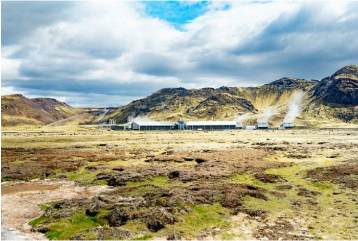
Hellisheidi Geothermal Power Station Landscape. Source: ON Power
