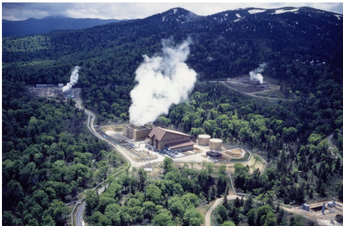
Sumikawa Geothermal Plant Aerial View.
