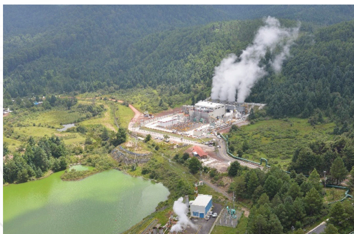
Aerial view of the Los Azufres geothermal power plant. Source: CFE
