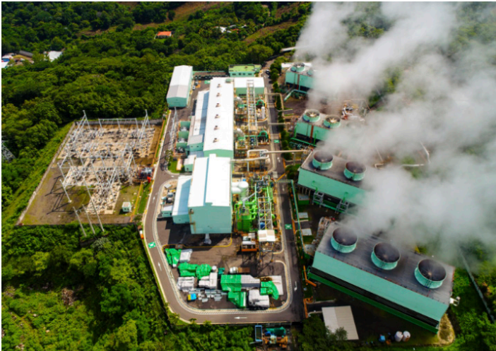
Berlin Geothermal Power Station, illustrating surface infrastructure. Source: LaGeo
