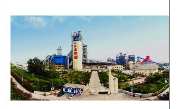
Linqu Shanshui Cement Co. , Ltd. has two new dry-process Rotary Kiln clinker production lines with a daily output of 4000 tons and a 16.5 mw pure low-temperature waste heat power plant and a cement grinding production line with an annual output of 1 million tons
